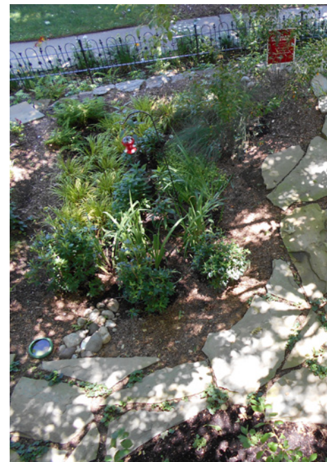
This shallow, planted depression absorbs the water that flows from a roof or patio.
