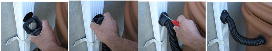
8. Double check to make sure all connections are secure. Provide winter cap to participant or leave on top of rain barrel. Make sure to leave correct version of winter cap (round or rectangular). Clean up debris (plastic shavings from barrel). Take “after” photo of the installation.
