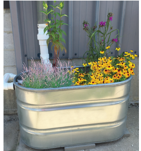
Connected to the roof downspout, these planters slow water down before entering the sewer while irrigating plants and removing pollutants.
