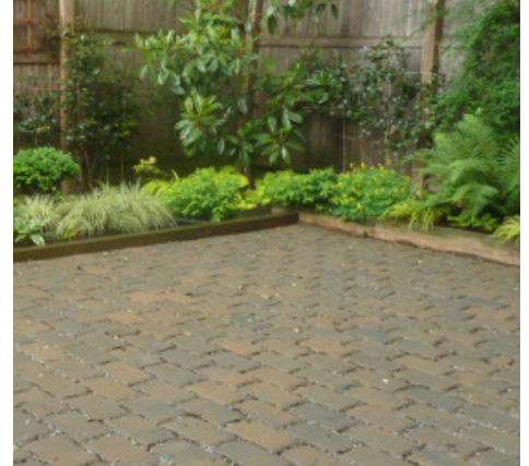
Permeable Pavers: Specially designed paving stones, bricks, or pavers that allow water to soak into the ground below.
