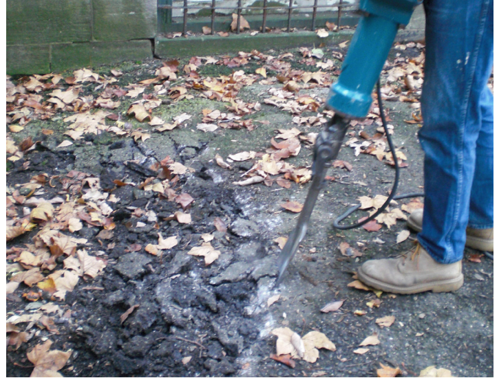
Depaving: The removal of concrete, asphalt or other impervious surfaces can provide space for a lawn, rain garden, clean stone or other landscaping.
