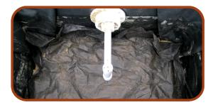
Place soil medium into planter to a height 1-2" below overflow drain inlet (atrium grate).
