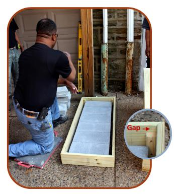
Use exterior grade composite shims (or other moisture-proof leveling material) to level the base. Shims should be placed to promote a fairly even distribution of weight. The base should be level in all directions.
