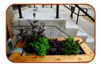
Place splash rock underneath the downspout diverter outlet to a depth of approximately 1" and covering around 1/3 of the soil. This will allow stormwater to disperse throughout the planter.
