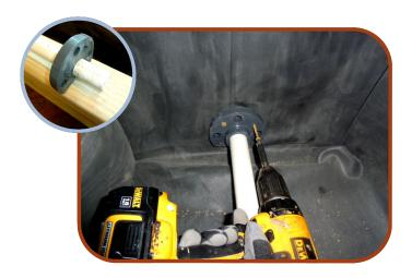
7. **Install Underdrain (continued).** Using PVC primer and cement, attach 1" 90 degree elbow to the other end of the PVC. Then, attach an 18" length of 1" PVC to the other part of the elbow for the vertical portion of the underdrain. Place 1" PVC slip cap on top of the vertical piece – do not glue – leave it removable for future cleanout. Attach 1" to ¾" threaded PVC adapter to the outlet end of the underdrain using primer and cement.
