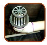
9. **Seal flanges.** Using latex gloves and roofing cement, cover both the underdrain and overflow flanges, creating a water barrier. Be careful not to get any roof cement on the outside of the planter or the trim. If you do, use paint thinner immediately to clean it. Seal penetrations at exterior using waterproof silicone and caulking gun.
